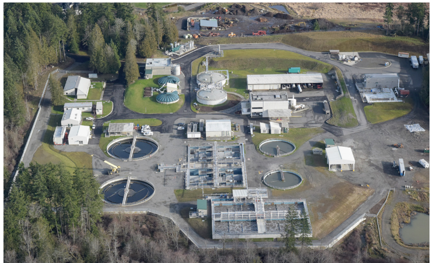
Central Kitsap Treatment Plant treats 3.5 million gallons of wastewater per day from Central Kitsap, Silverdale, Keyport, Bangor Naval Base, Naval Undersea Warfare Center, and the City of Poulsbo.
