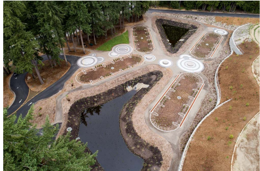
Whispering Firs Stormwater Park, Silverdale, WA Photo Courtesy: Michele Filley, Kitsap County Public Works
