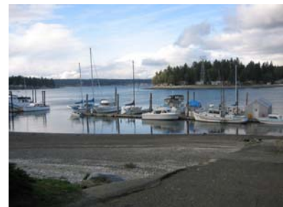
Figure 6.3.1 Port of Keyport Dock
