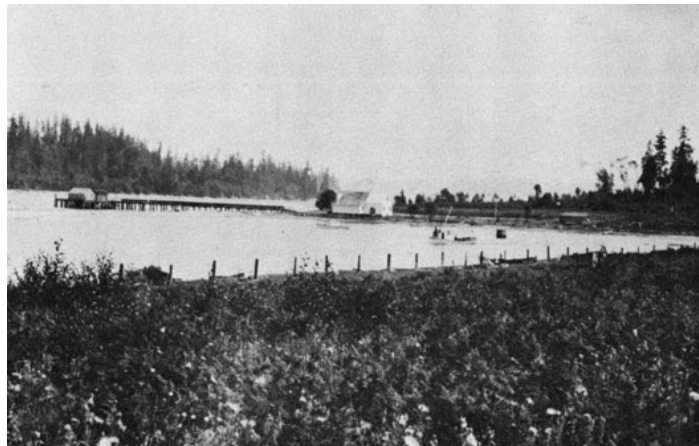
Figure 5.1.3 Original Keyport Store & Community Dock.
