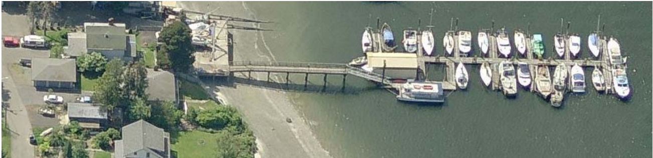
Figure 5.2.1 Keyport Marine Services facilities.
