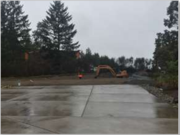
Industrial Park Site Under construction (1/9/2020)
