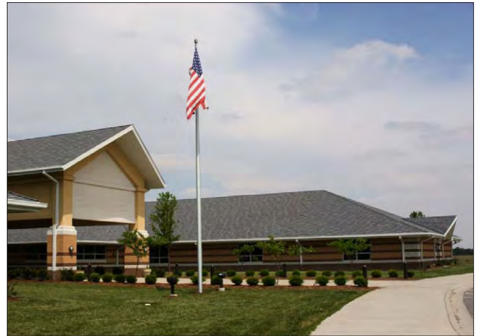
K-12 schools represent a highly vulnerable use and should be prohibited near airports.
