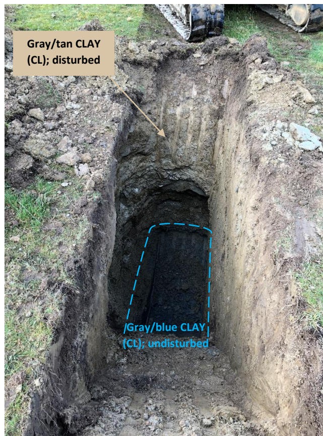
Photo 2: Subsurface conditions encountered in TP-1.
