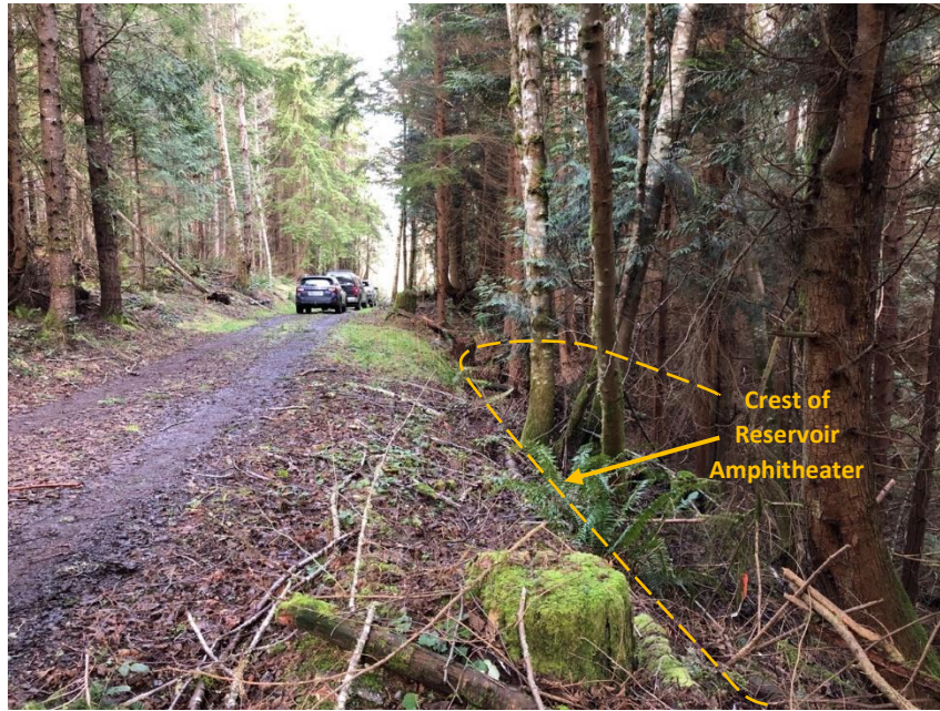
Photo 9: View facing north along access road near the crest of the reservoir amphitheater.
