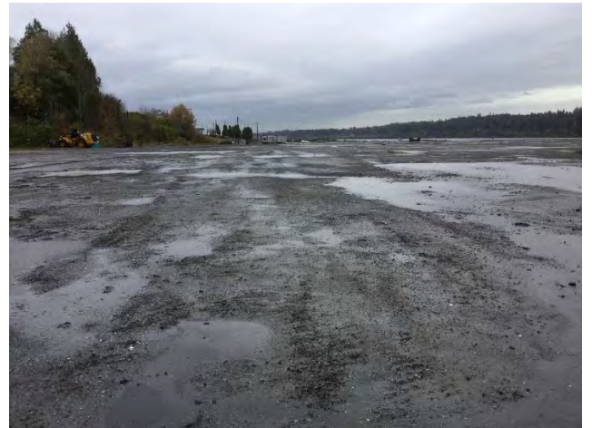
Photograph 12. Looking north across the south end of the cleanup site.
