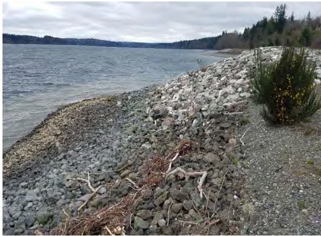
Photograph 11. Typical shoreline post clean-up with sparse invasive species, armor rock and cobbled beach.
