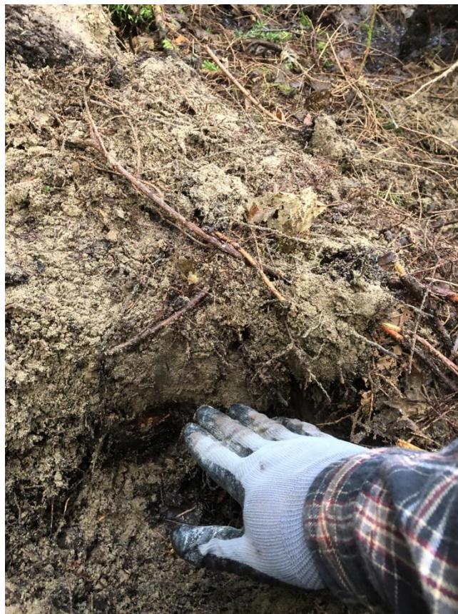
Photo 12: Shallow handholes encountered loose, fine to medium sand within and around the reservoir amphitheater.
