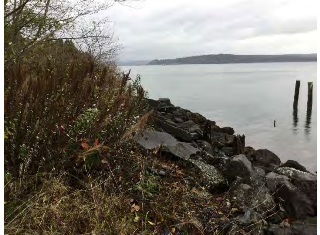
Photograph 2. Looking north along the shoreline in the northern Mill Site area. The shoreline in this area is covered in riprap, concrete and asphalt chunks and has a small vegetated buffer.
