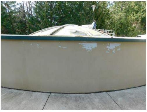
Loss of top coat, no associated rust staining or corrosion
