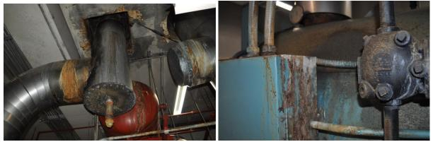
Figure 3 – Rusty Boiler Components due to the Leaking Roof Penetrations
