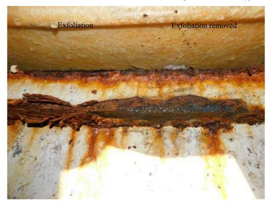
Corrosion of stiffener channel
