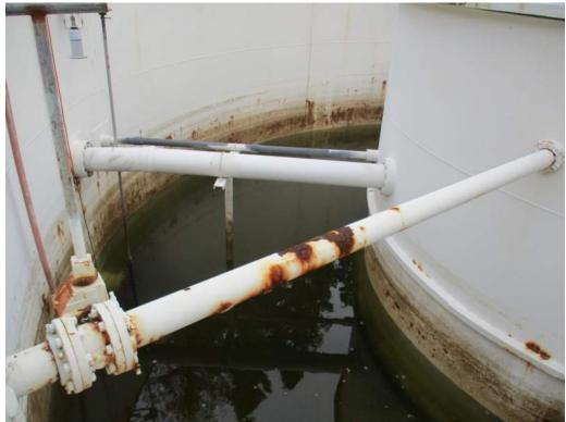
Photo 3 – Corrosion of Piping at the EQ Basin
