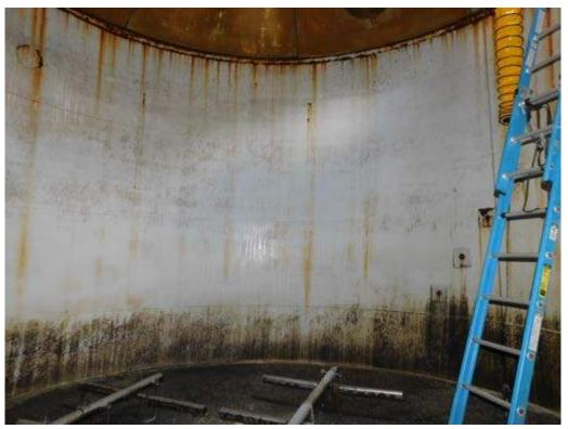
Sludge tank interior sidewall, typical coating, and corrosion condition
