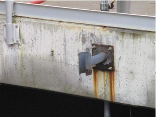
Photo 5 – Corrosion of Metal Plate at SBR Basins
