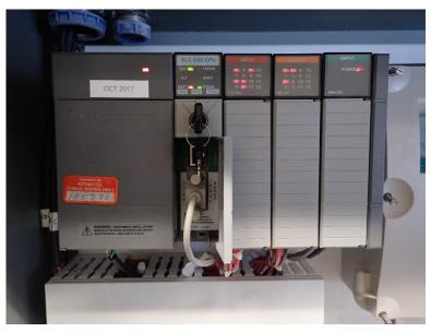
Another observation is that the RIO control panel in the MWWTP blower building is installed above the old SBR control panel and is not readily accessible. Figure 3-4 shows this panel with its door open above the SBR control panel. Sewer Utility staff would need a ladder to perform modifications to the panel or troubleshoot its wiring.
