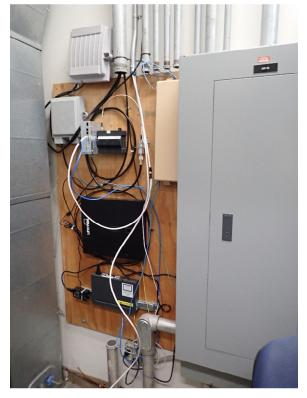
The Sewer Utility has implemented a separate Internet service for the MWWTP business LAN, which consists primarily of a wireless access point and a laptop located in the operations building control room. Internet access for the business LAN is achieved via a Motorola SB5120 cable modem. HDR did not review configuration or security settings for this device.
