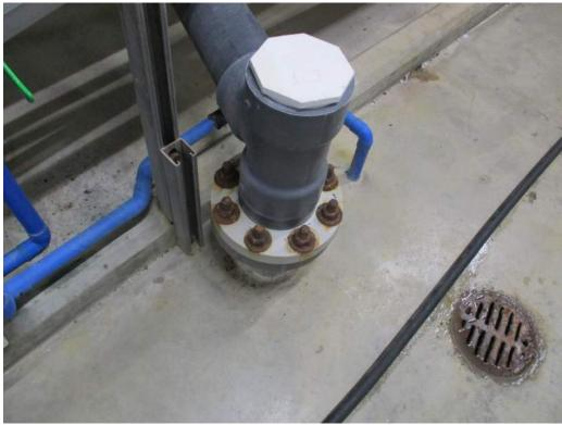
Photo 9 – Bolt Corrosion at Process Building (Upper Floor)
