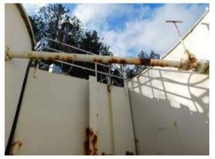
Coating losses on bottom of piping
