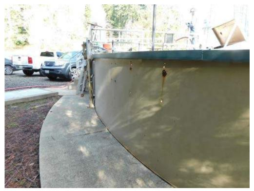
Coating damage at wall penetrations
