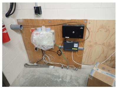
The Sewer Utility has implemented a separate Internet service for the KWWTP business LAN, which consists primarily of a PC located in the operations building control room. Internet access for the business LAN is achieved via a Peplink PEPWAVE MAX BR1 mini-cellular router. HDR did not review configuration or security settings for this device.
