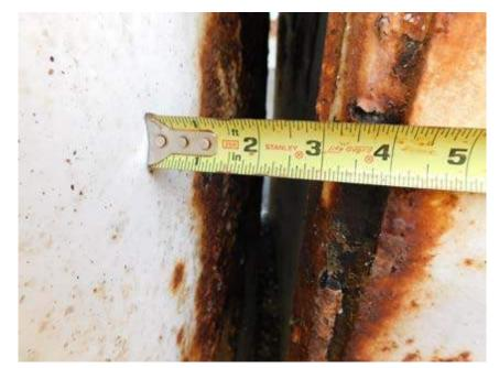
Gap between sidewall and chamber transition, inaccessible for inspection and coating upgrades
