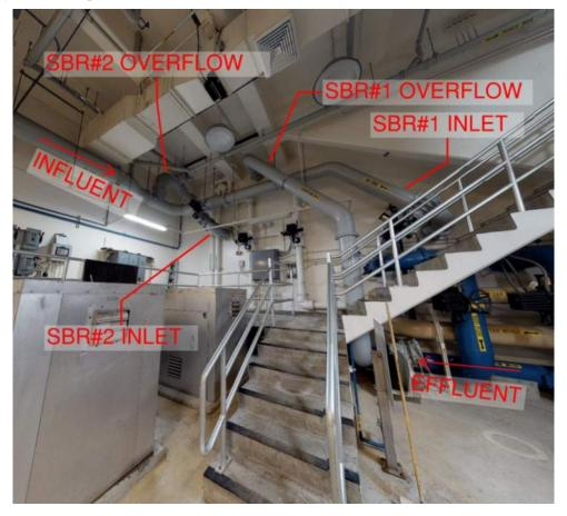
Figure 3-3 | Overflow Pipe
