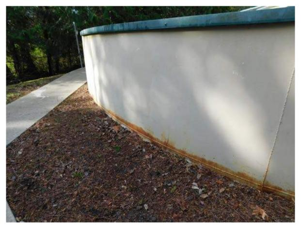
Surface rusting at soil-to air interface, no pitting observed
