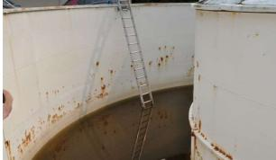
Equalization basin piping and corrosion
