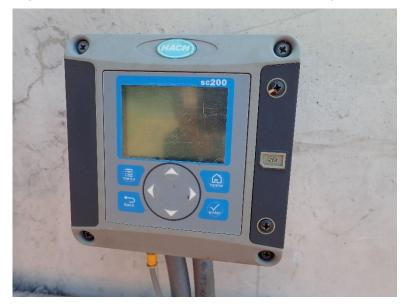
Figure 3-17. CKTP reclaimed-water filtration system turbidity analyzer powered down
