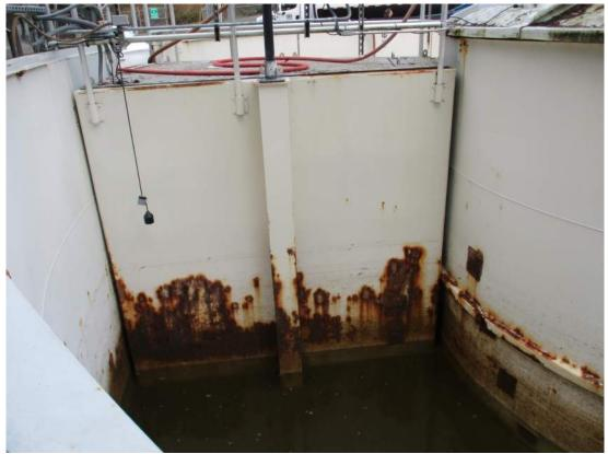
Photo 2 – Corrosion at the EQ Basin
