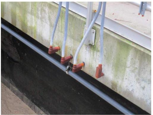
Photo 6 – Corrosion of Metals at SBR Basins
