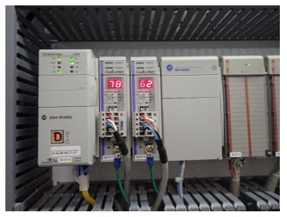
Figure 3-5. DeviceNet scanners in PNL 2939 PLC rack
