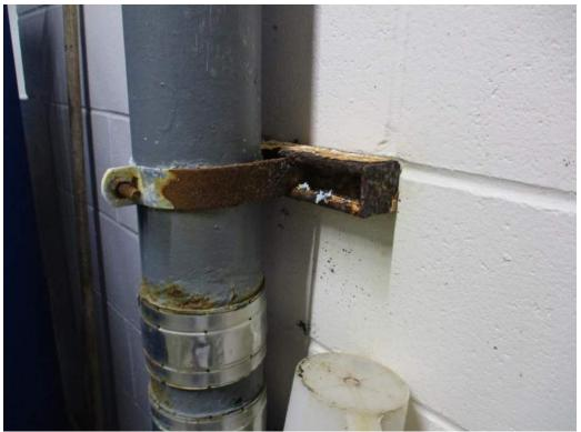
Photo 8 – Corrosion of Metal Component in Process Building (Upper Floor)
