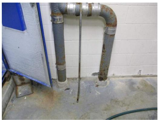
Photo 7 – Corrosion of Metal Pipes in Process Building (Upper Floor)
