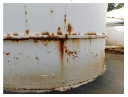
Lower surface of sludge tank, corrosion at stiffener channel
