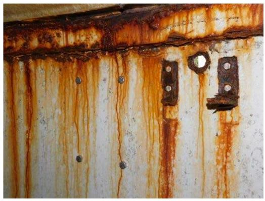
Corrosion of stiffener channel installed around the inner perimeter of tank, typical
