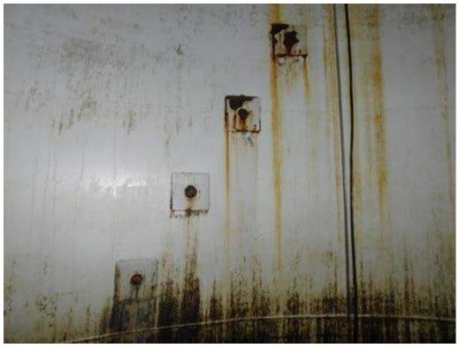
Weld patches – coating loss and surface corrosion
