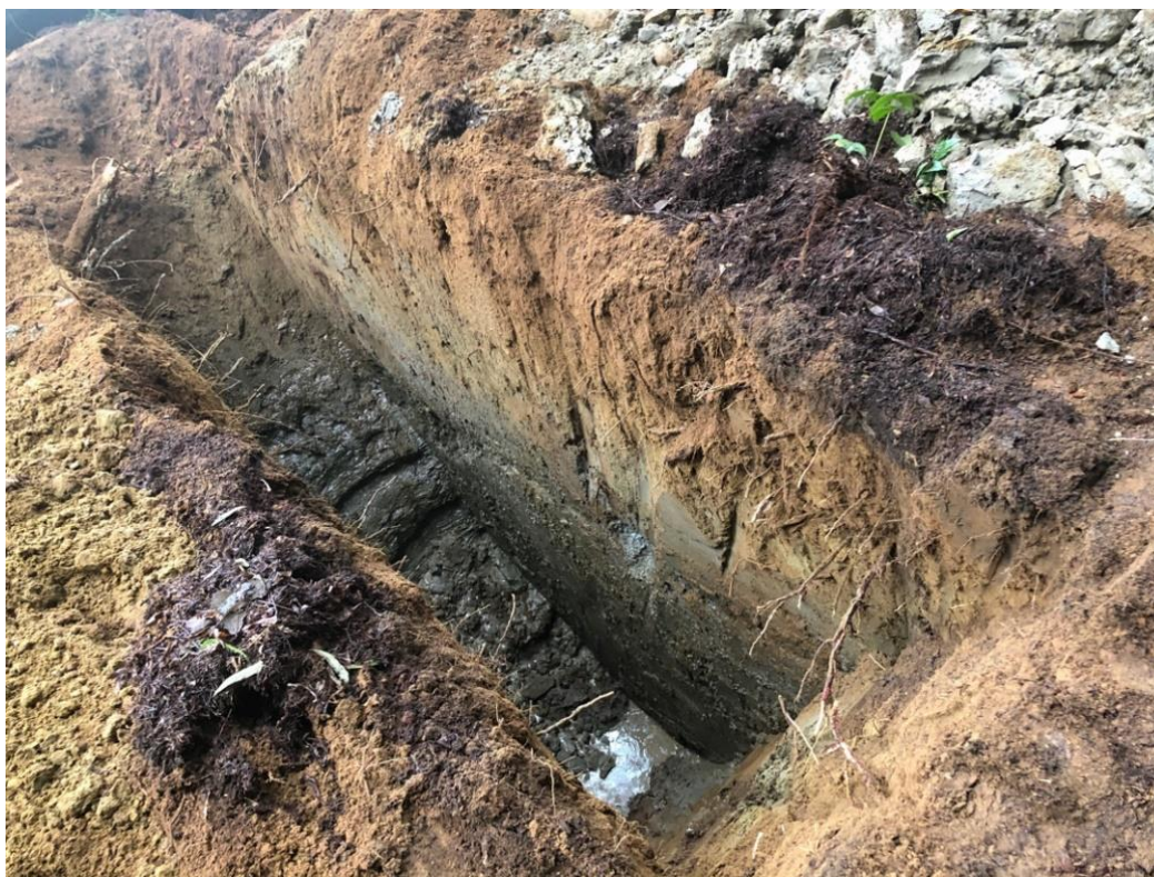
Photograph 3. Test Pit ATP-02; showing groundwater seepage into the pit.
