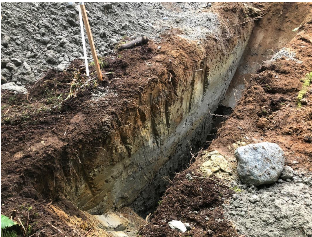
Photograph 2. Test Pit ATP-03; showing transition from highly weathered Vashon till to weathered Vashon till.
