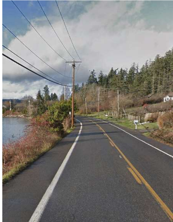
Picture 4 – Lemolo Shore Drive NE west of Peterson Way NE
