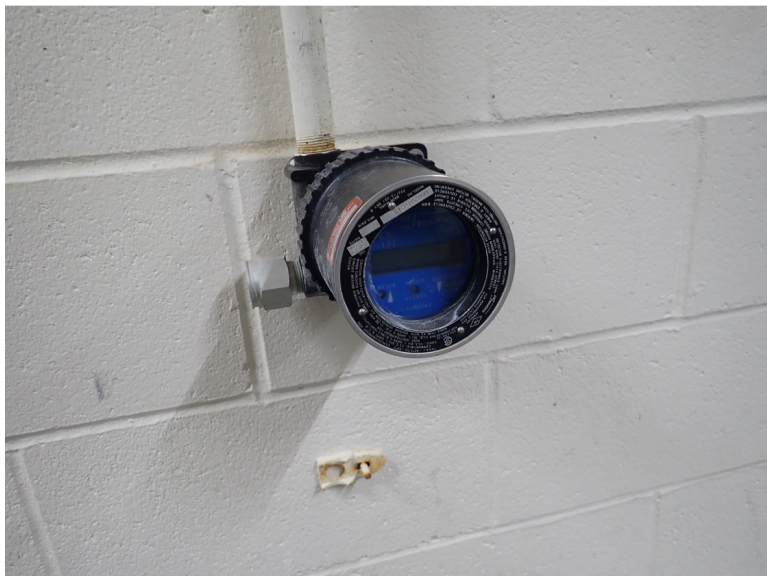
Figure 3-24. Non-functional LEL gas monitor in the SWWTP process building upper-floor process room
