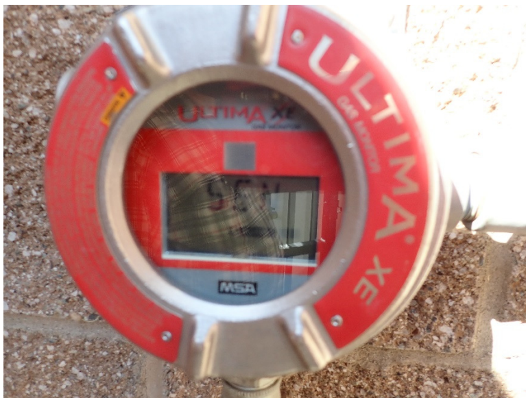
Figure 3-33. PS-71 wet well LEL monitor in alarm
