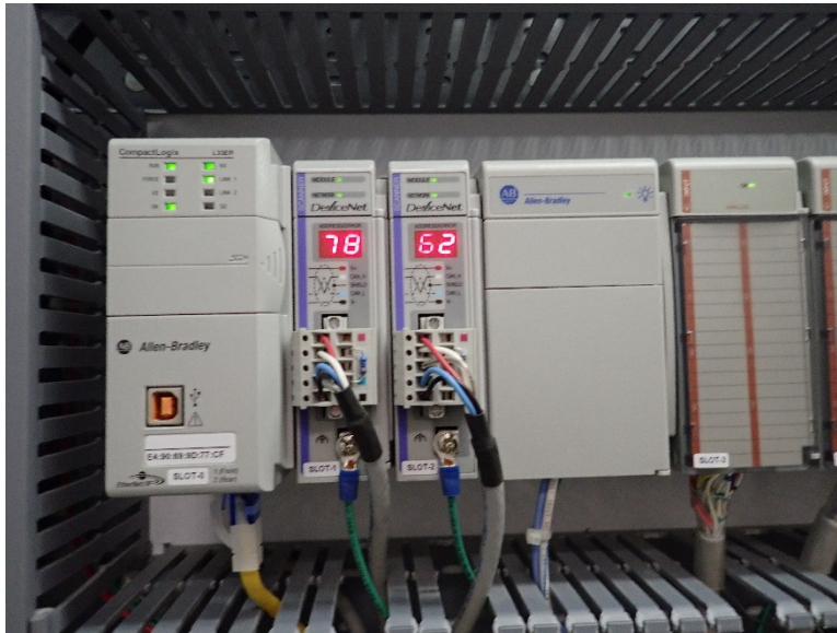
Figure 3-5. DeviceNet scanners in PNL 2939 PLC rack
