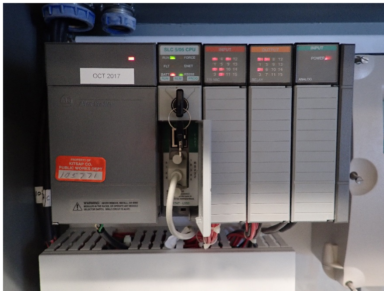
Figure 3-3. CKTP bar screen 1023 main control panel PLC controller battery alarm light illuminated
