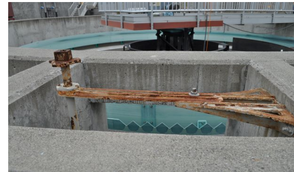
Clarifier effluent box valve stem
