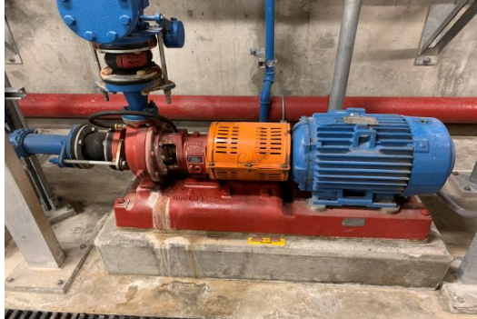
P-902 W32 Pump gasket leak
