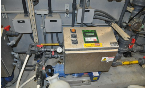
P-811 Polymer Metering Pump
