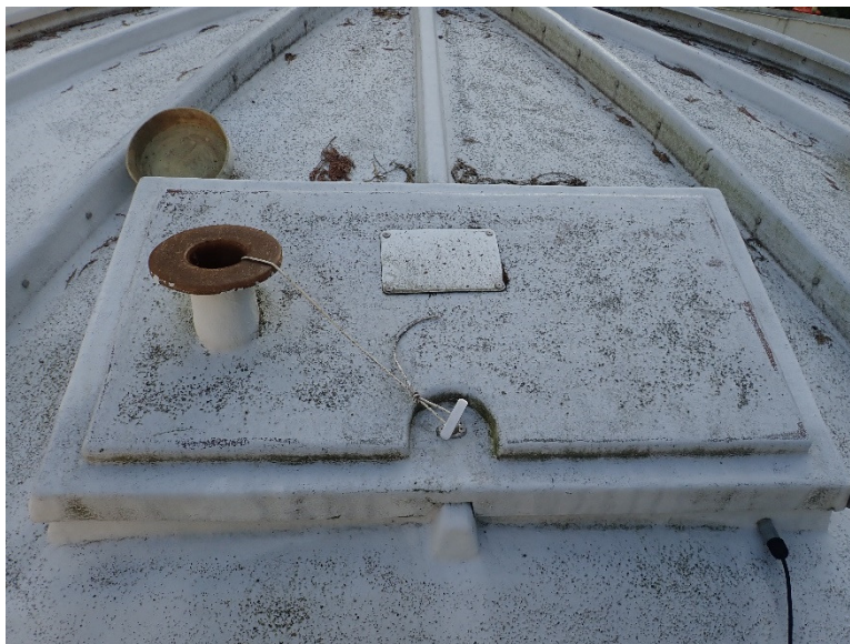
Figure 3-26. SWWTP sludge storage tank high-level switch installation
