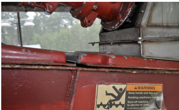
Corrosion on M-205 Grit Cyclone and Classifier
