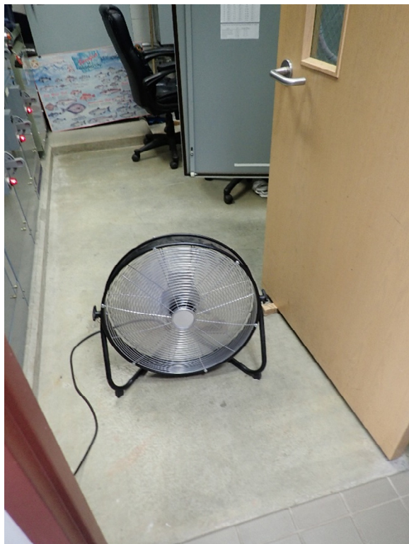
Figure 3-9. Temporary ventilation measure for MWWTP electrical room
