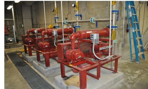
B-601-3 Sludge Tank Blowers
