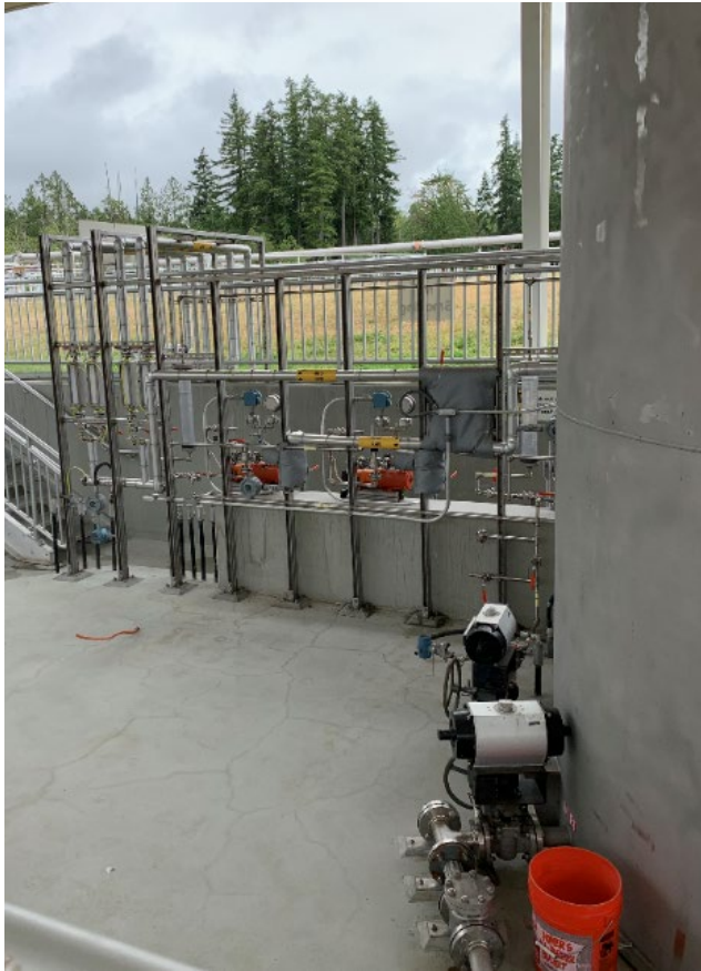
Figure 3-6. Existing CKTP methanol storage and feed system
