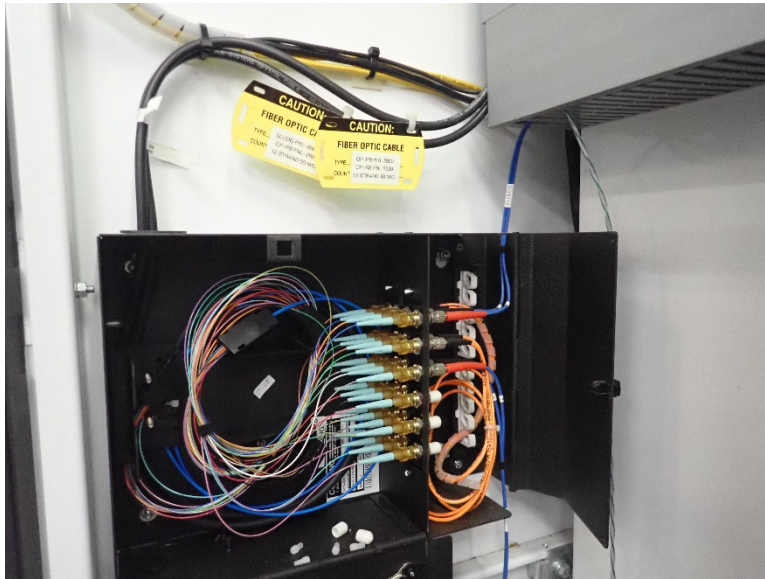
Figure 2-9. OM1 patch cord used to patch OM3 cables in PNL 2920
