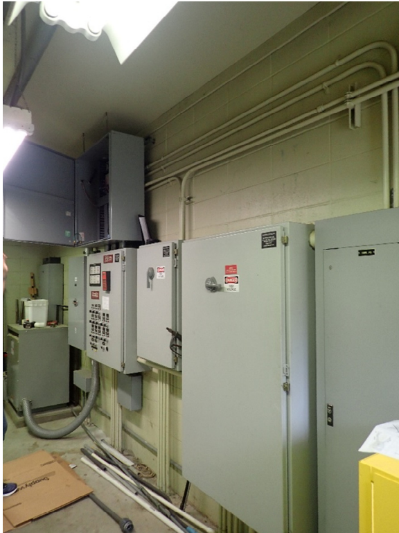
Figure 3-4. MWWTP blower building RIO control panel installation
