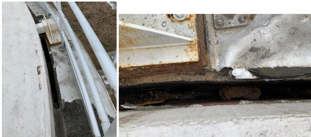
Figure 1 – CKTP Digester 2 Seal Failure
