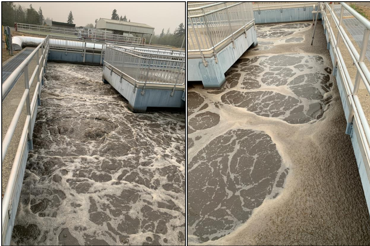
Figure 2 Coarse Bubbles from Failed Strip (Left) and Fine Bubbles from Functional Strip (Right)
