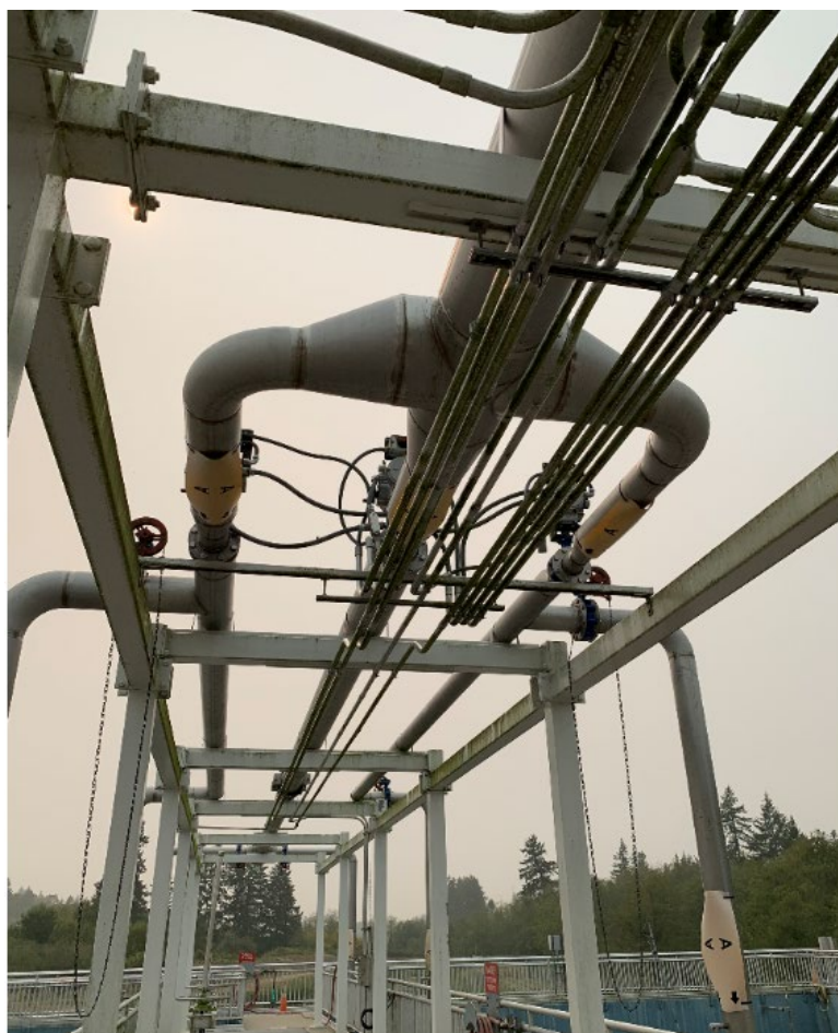
Figure 3-4. Typical aeration control piping for basins (three branches, each with a control valve, routed to a pair of zones with manual drop legs)
