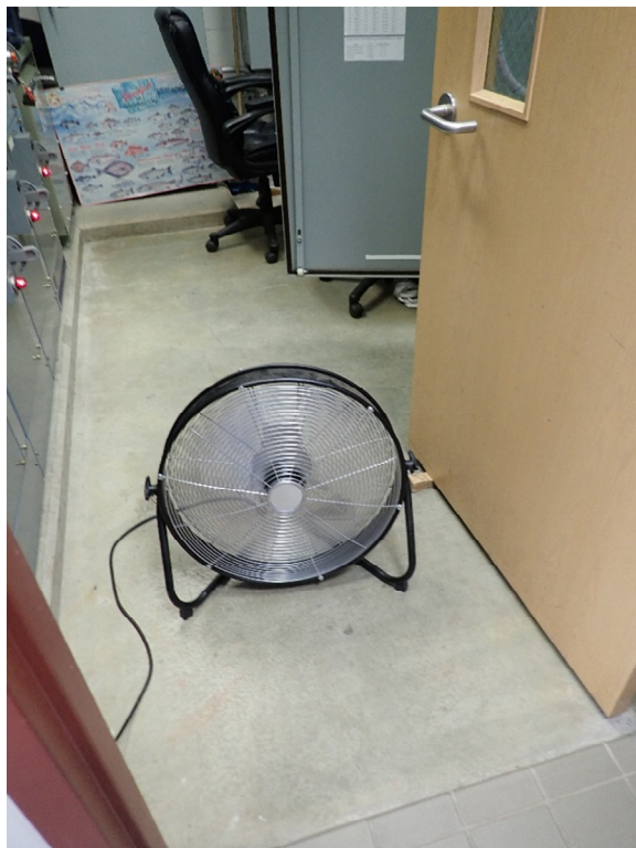
Figure 3-9. Temporary ventilation measure for MWWTP electrical room
