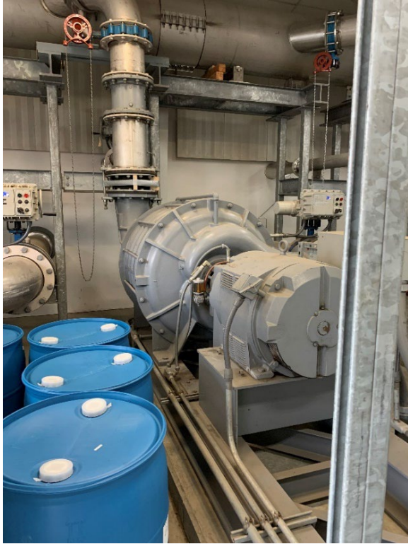
Figure 3-11. Example Lamson multistage centrifugal blower
