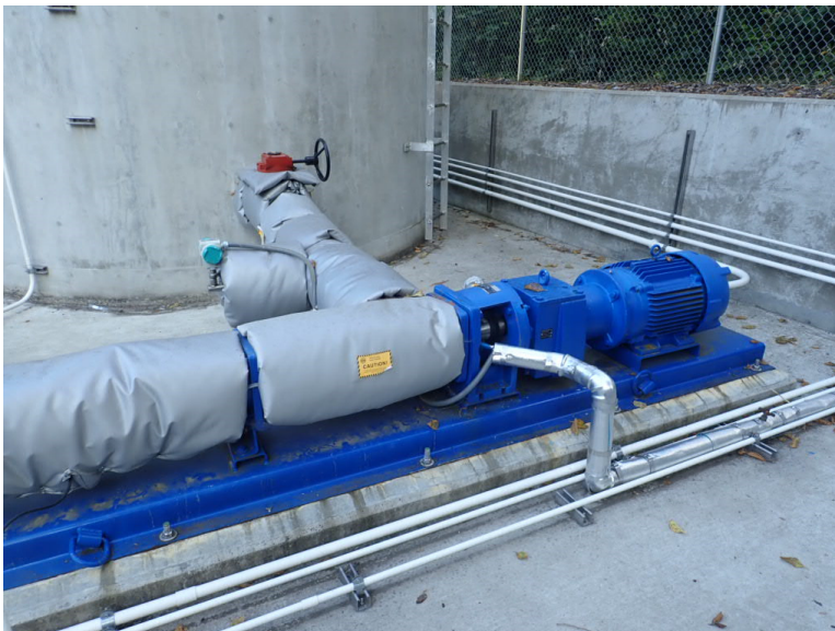
Figure 3-25. SWWTP thickened sludge tank level transmitter on truck loadout pump suction piping
