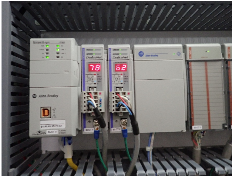
Figure 3-5. DeviceNet scanners in PNL 2939 PLC rack
