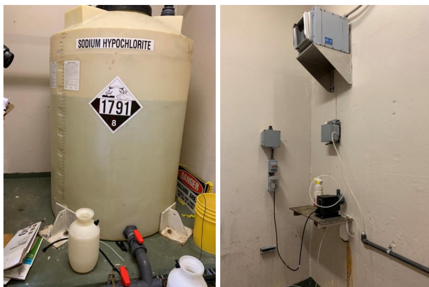
Figure 4 – MTP Sodium Hypochlorite Storage Room
