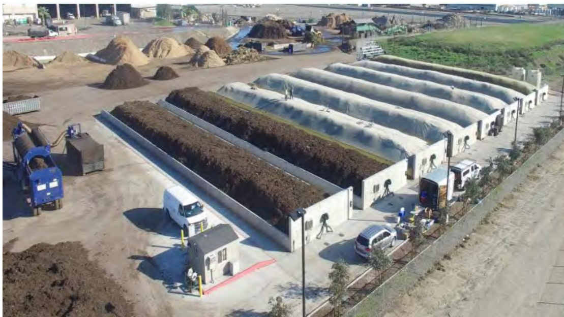
Figure 8-7 | Static Aerated Pile Composting Facility
