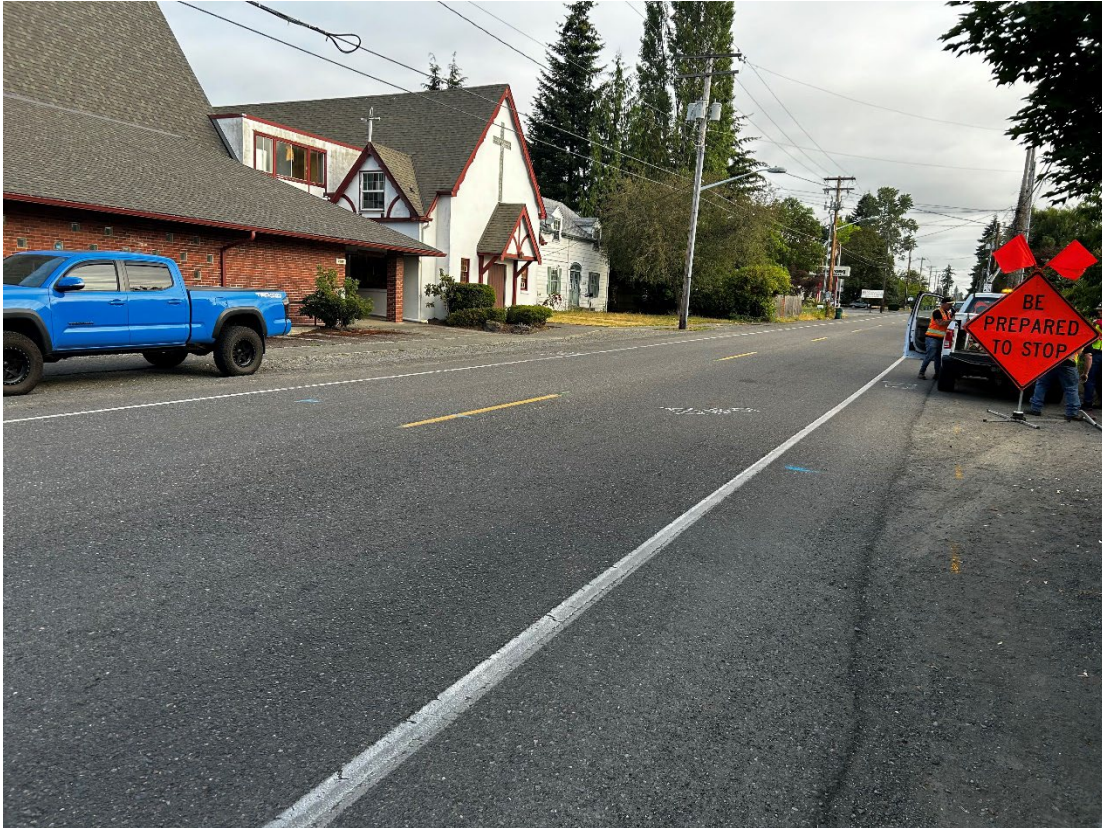
Photograph 1. Perry Avenue NE, looking north near AB-01 at representative pavement conditions.
