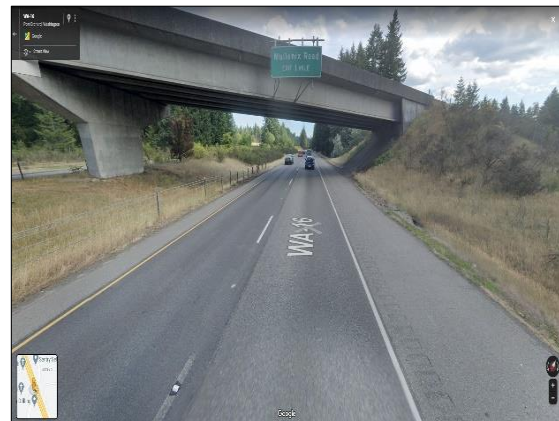
Southbound State Hwy 16 below Bethel-Burley overpass
