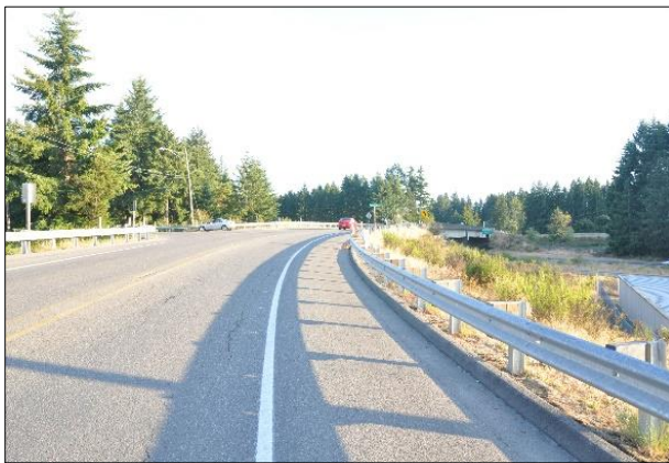
Southbound Bethel-Burley Rd SE
