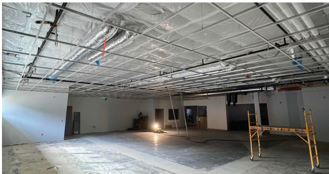
Installation of the ceiling grid and interior painting
