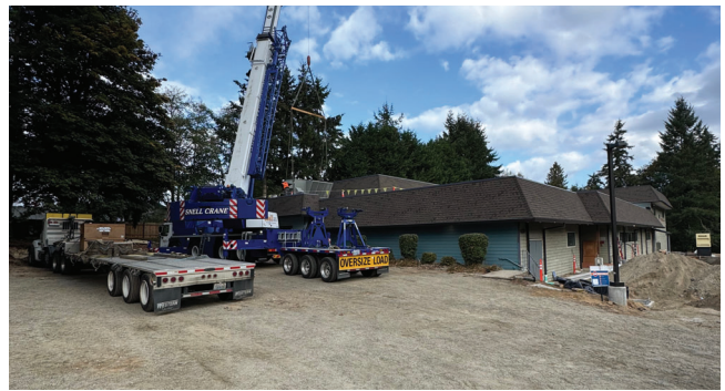
HVAC unit delivery
