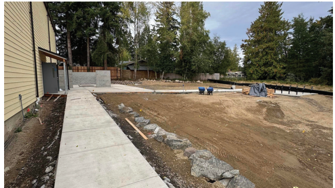
HVAC enclosure and concrete work
