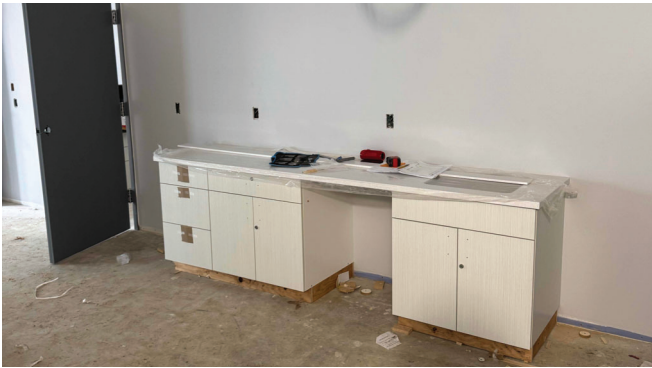
Cabinets and countertops installed
