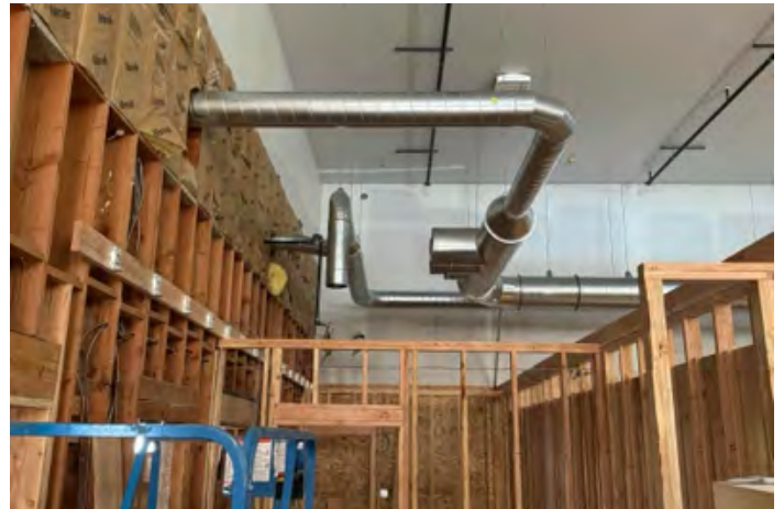
HVAC ductwork Installation
