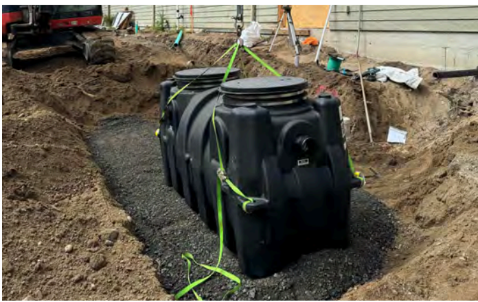
Grease interceptor installation
