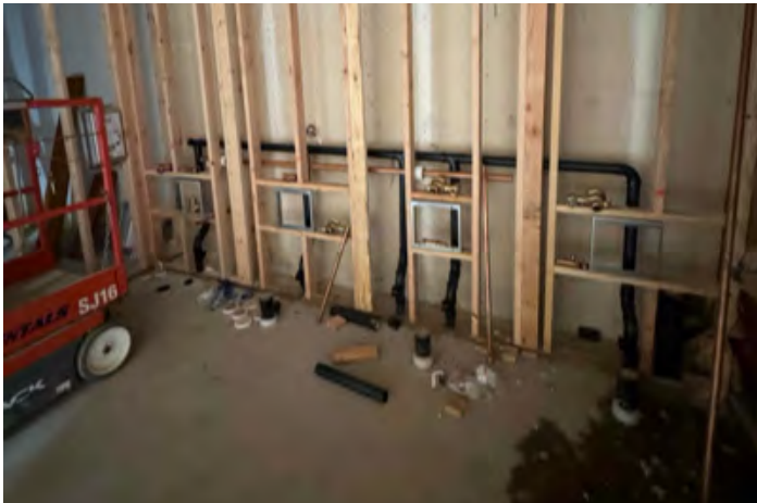
Bathroom plumbing rough-in
