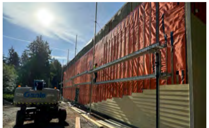
Siding installation
