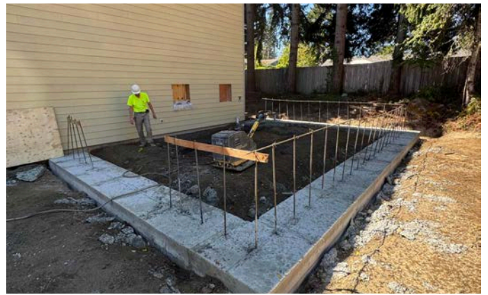
Concrete Footings for the HVAC slab
