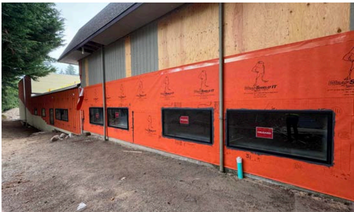
Completed Exterior Window Installation
