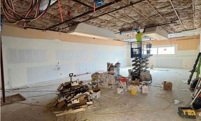
Insulation and Drywall Installed
