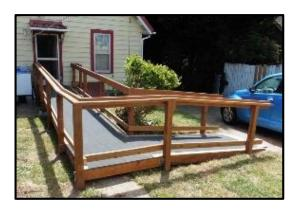
Ramps are custom built using pressure treated (weather resistant) lumber. They can be straight, L-shaped, or switchback to fit the site.
