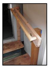
This simple, low cost handrail provides a sturdy gripping surface.
