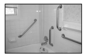
Grab bars on the shower/tub wall can help a person safely lower themselves onto a seat or into the water, and make getting out much safer.
