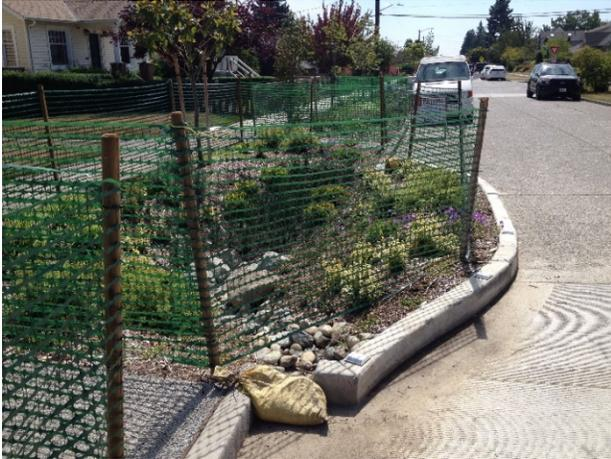
*Sand bags prevent silt-laden flow from entering the bioretention BMP. Green construction fencing prevents compaction due to foot traffic.*
