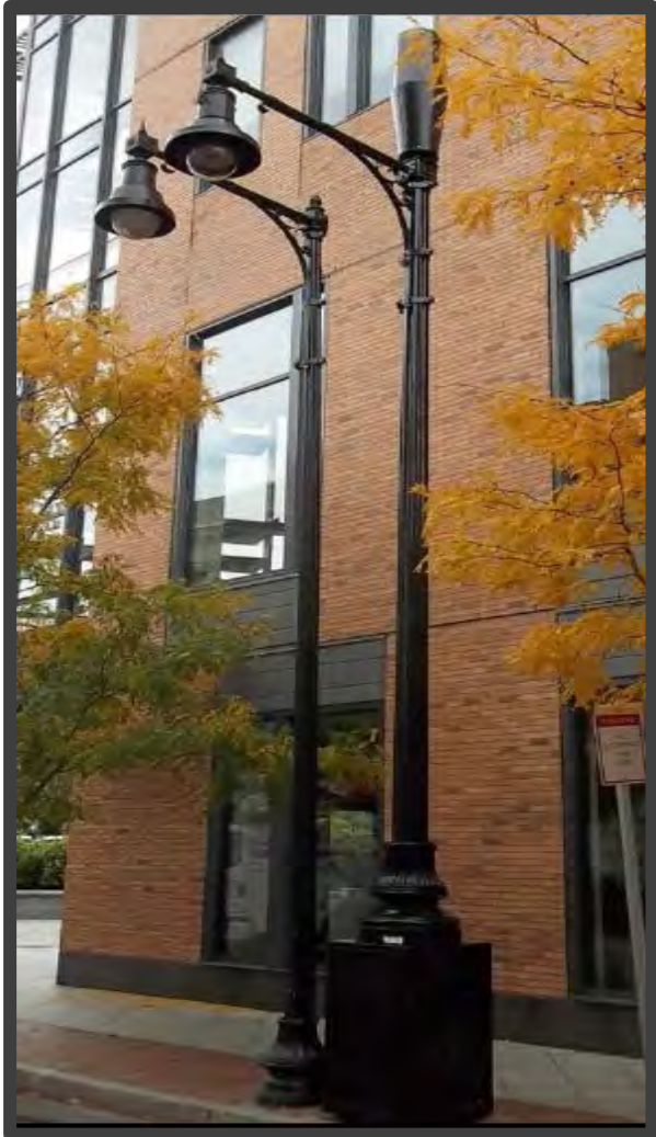
New small cell decorative pole next to existing pole before removal.
