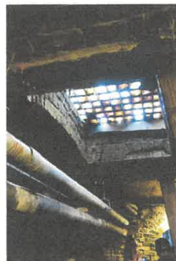
A view looking upwards at the vault lights (glass skywalks). The roof of a building at previous street level; now the top of the glass is walked upon and forms the current sidewalk.
