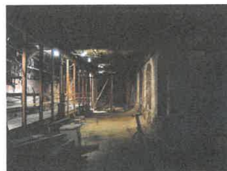
The concrete floor of the former meat market was originally at the level of the wooden platform on the left but sank over time because of decomposing sawdust fill.
