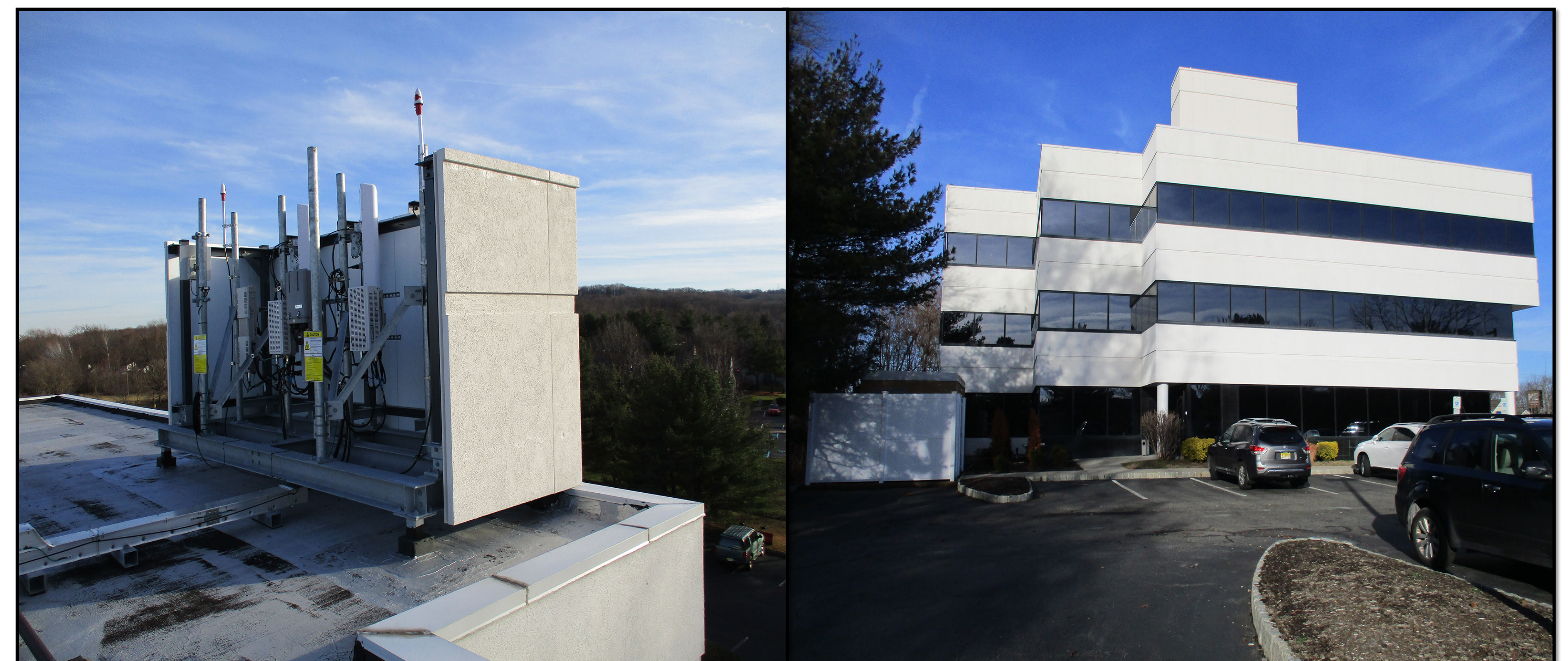
Image Source: http://fcarchitectsinc.com/services/traditional-facilities/#iLightbox/gallery_image_2/0
