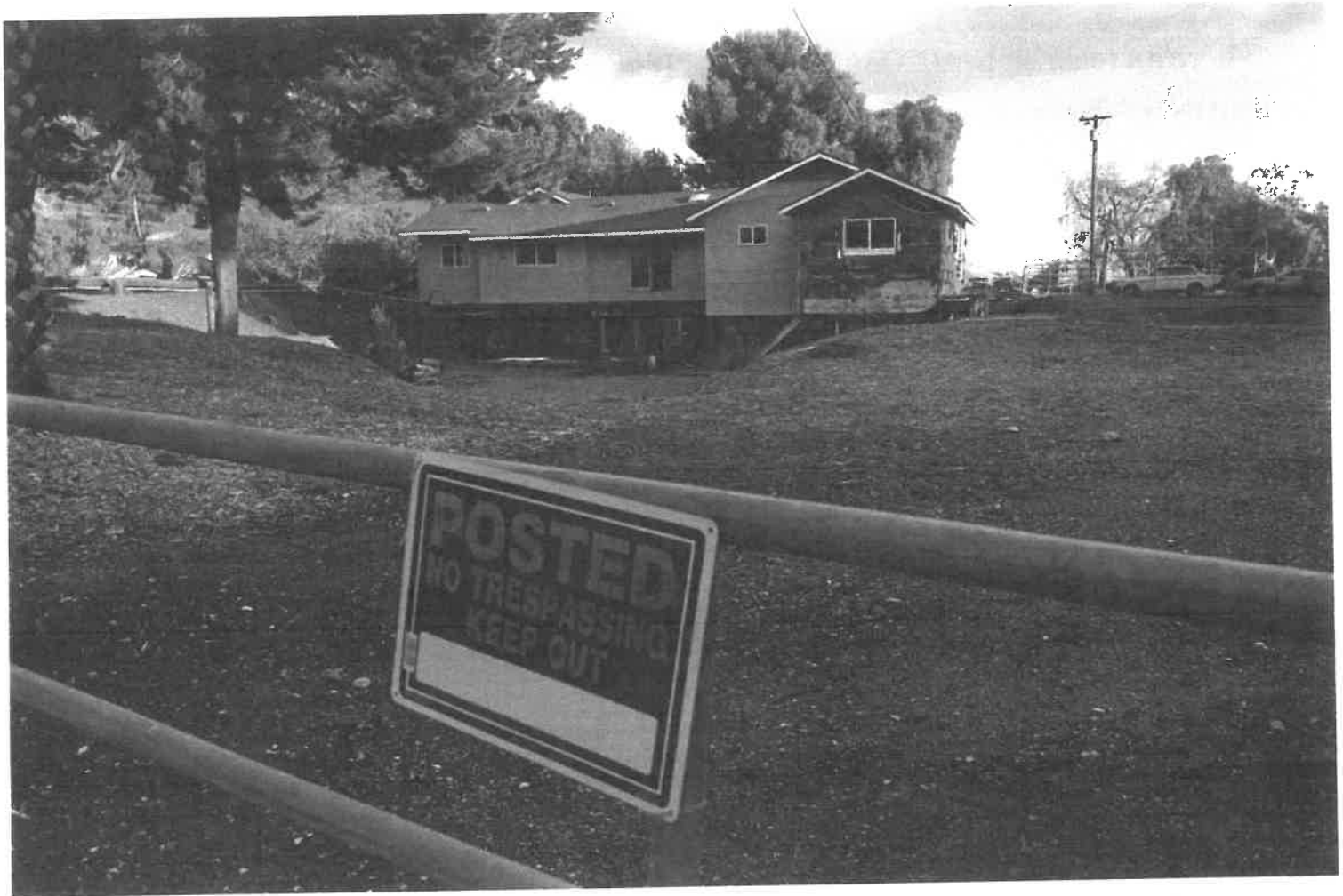
Some houses in Portuguese Bend are propped up on timber cribbing to keep the foundation steady with the shifting land. (Carolyn Cole / Los Angeles Times)
