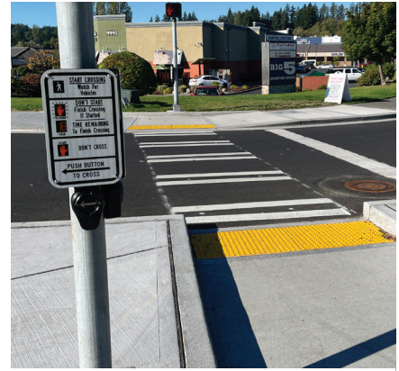
Figure 6.33 Pedestrian safety infrastructure on Silverdale Way
