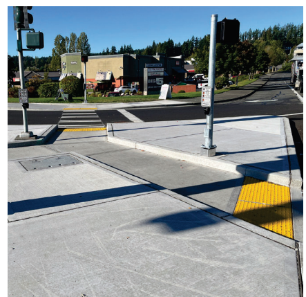
Figure 6.27 Improvements to pedestrian infrastructure on Silverdale Way
