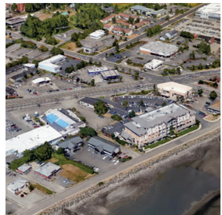
Figure 3.11 Without a clear plan for building community, Silverdale’s land uses and urban form have developed in a fragmented, disconnected way
