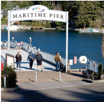
Figure 6.12 Maritime Pier, Gig Harbor
