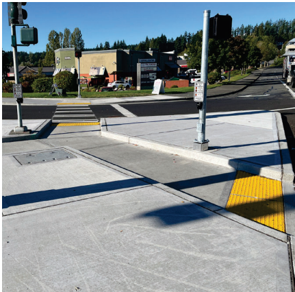
Figure 6.27 Improvements to pedestrian infrastructure on Silverdale Way
