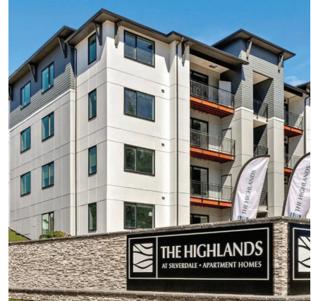
Figure 1.6 The Highlands - Recent multifamily construction example just outside (north) of the Silverdale Regional Center Boundary
