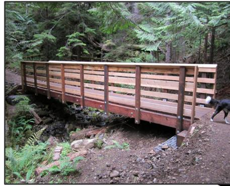
Timber Bridge Example (5 ft. wide, grating tread, glu-lam beams)
