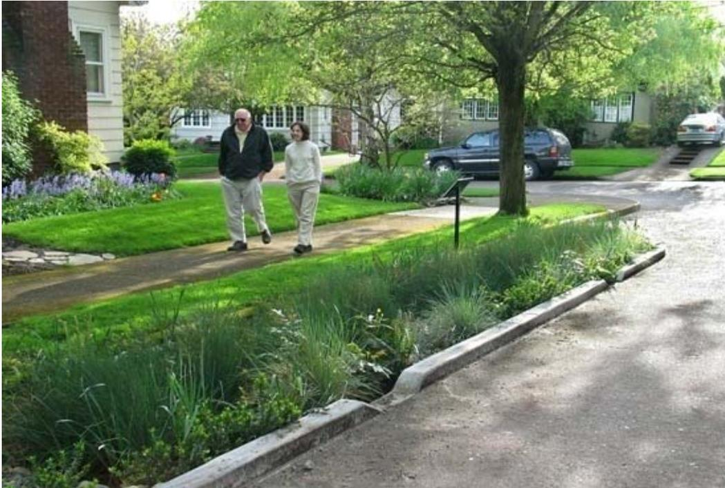
*Figure 14.4: Siskiyou project in Portland, Oregon uses traffic calming designs to manage stormwater. Note curb cuts that allow stormwater to enter bioretention area in narrow section of road.*
