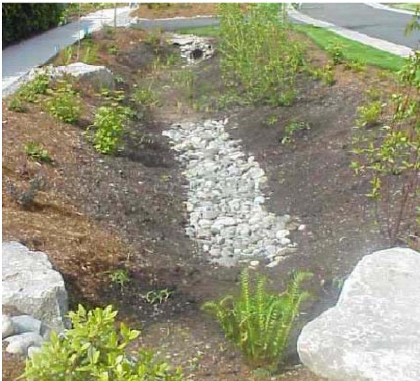
*Figure 14.3: Seattle SEASStreets bioretention swale receiving sheet flow from sidewalk and street*
