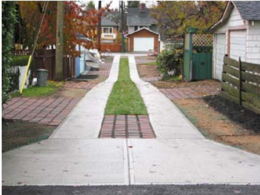
*Figure 19.1: Country Lane Alley in Vancouver, B.C. uses a combination of concrete wheel strips, pervious pavers, reinforced plastic grid with grass, and under-drains to attenuate storm flows and create an aesthetic design objective. Photo by Curtis Hinman*
