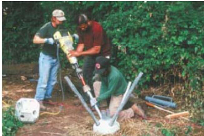
*Figure 20.3: Using an automatic hammer to pound pins.*
