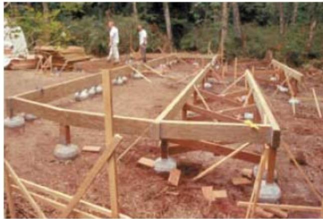
*Figure 20.2: A house construction project using minimal excavation foundation pier system.*
