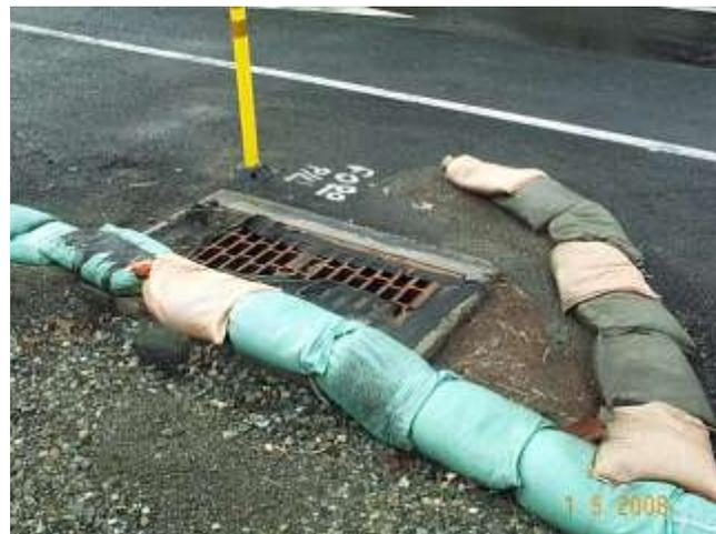
*Temporary sand bags divert construction site stormwater runoff to inlet protected with filter fabric.*
