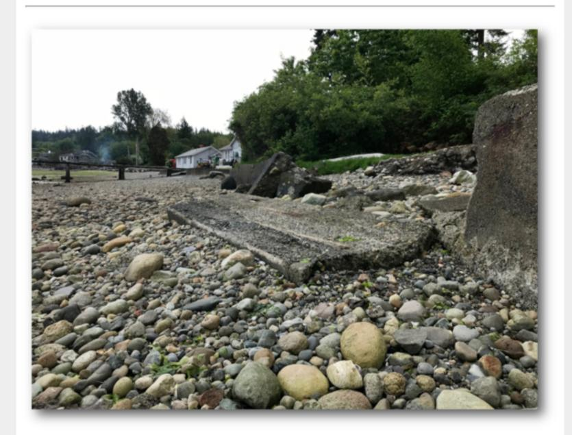
This picture shows a concrete bulkhead in Yukon Harbor. This bulkhead partially collapsed due to the loss of beach sand. Notice how the beach is made up of lots of large cobble and not much sand.
