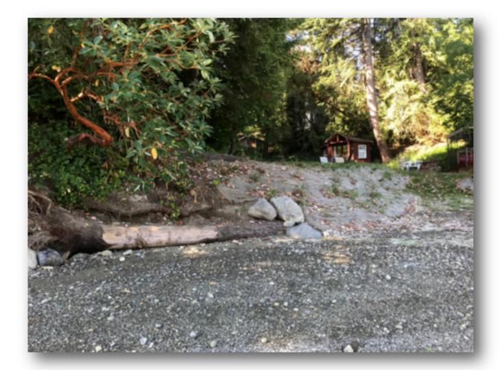
Oyster Bay soft-shore/restoration project. Fifty feet of wooden bulkhead were removed, and a log and plants were installed for soft-shore protection.
