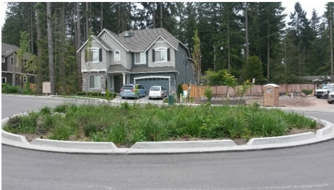
Bioretention in a cul-de-sac of an LID residential neighborhood in construction in western WA. The bioretention manages stormwater runoff from the roadway and contributing roof and driveway areas. Numerous large existing trees were retained, adding valuable stormwater and community benefits.
