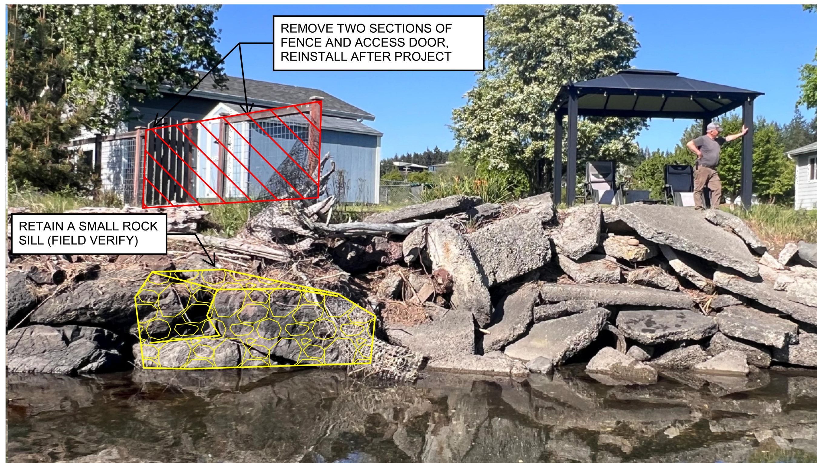
B ROCK SILL AT SECTION B (ILLUSTRATION ONLY, NOT TO SCALE)
