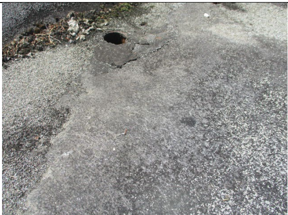
Drain in upper roof
