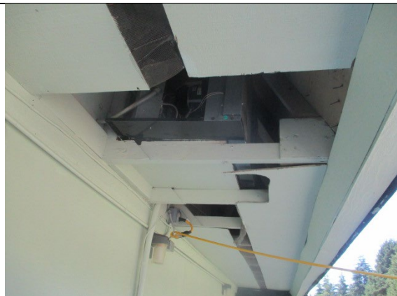
Open soffit on west side
