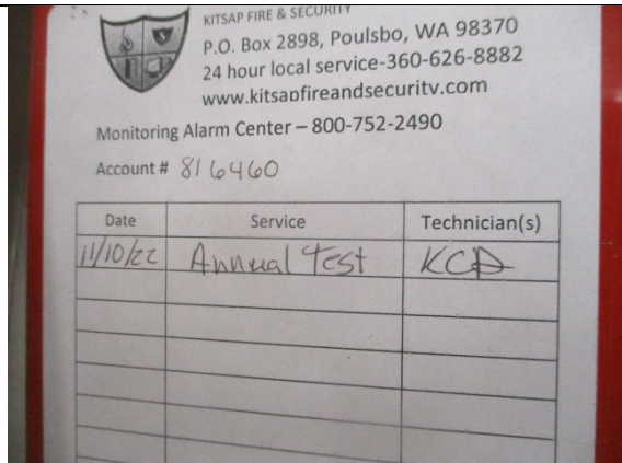
Service tag on alarm system
