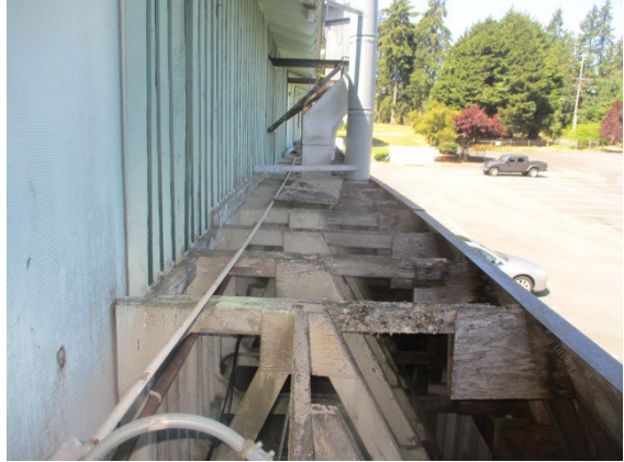
Open top of screen wall and mansard roof
