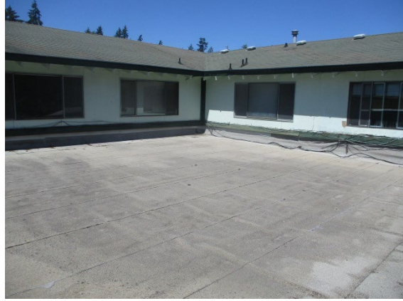
Overview of upper flat roof
