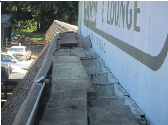
Open area at top of screen wall
