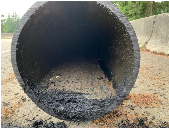
Figure 4-1. 18-inch Bypass Pipe
