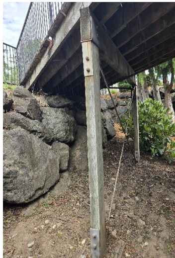
Figure 3: Ramp support & metal fencing
