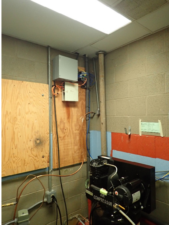
Figure 2-24. Exposed plumbing next to network components in CKTP administration and lab building electrical room
