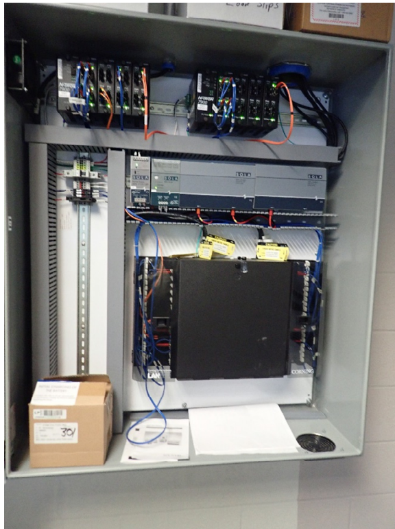
Figure 2-3. Modular access switches in PNL 8580A
