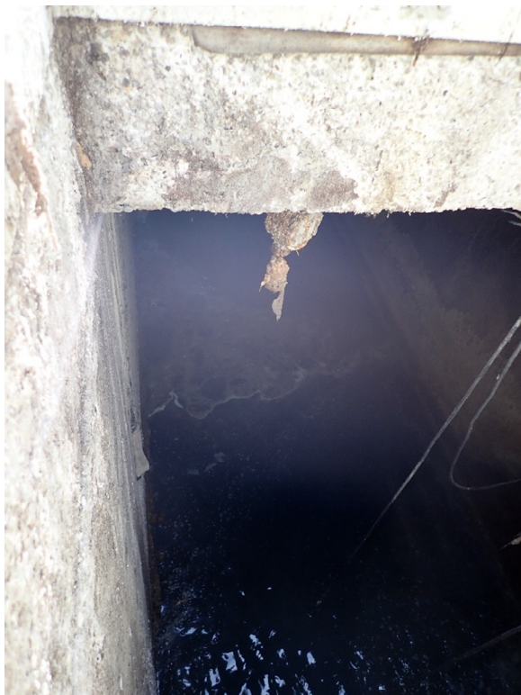
Figure 3-30. PS-24 wet well ultrasonic level transducer coated with grime and dried scum
