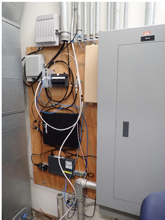
Figure 2-18. MWWTP operations building electrical room communications backboard
