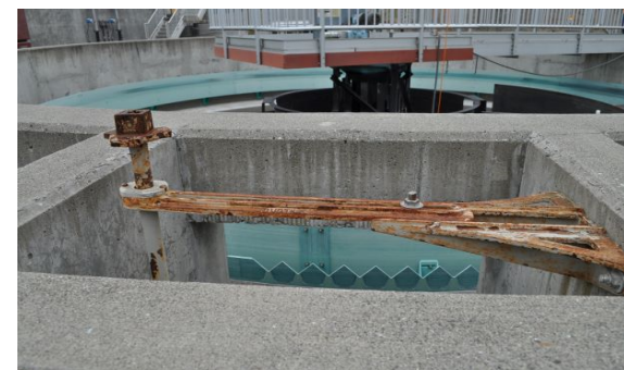
Clarifier effluent box valve stem
