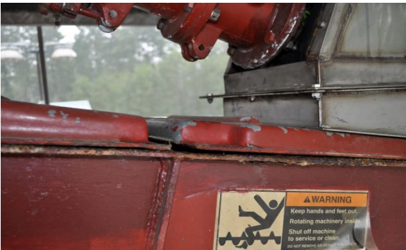
Corrosion on M-205 Grit Cyclone and Classifier
