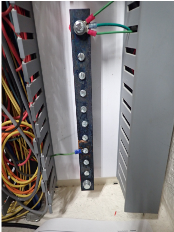
Figure 3-7. H_2S corrosion on digester control building control panel (PNL 6000) copper ground bar
