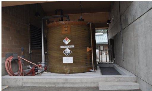
T-810 Sodium Hydrochlorite Tank
