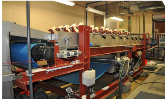
M-615 Gravity Belt Thickener
