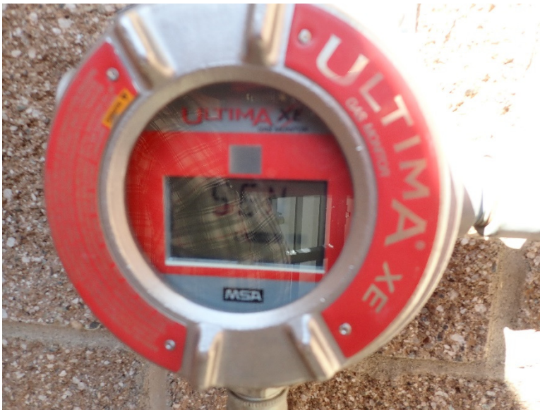
Figure 3-33. PS-71 wet well LEL monitor in alarm
