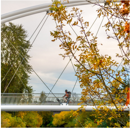
Figure 6.31 Tukwila Urban Center Bridge
